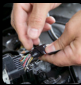
Repairs/insulates electrical wires
